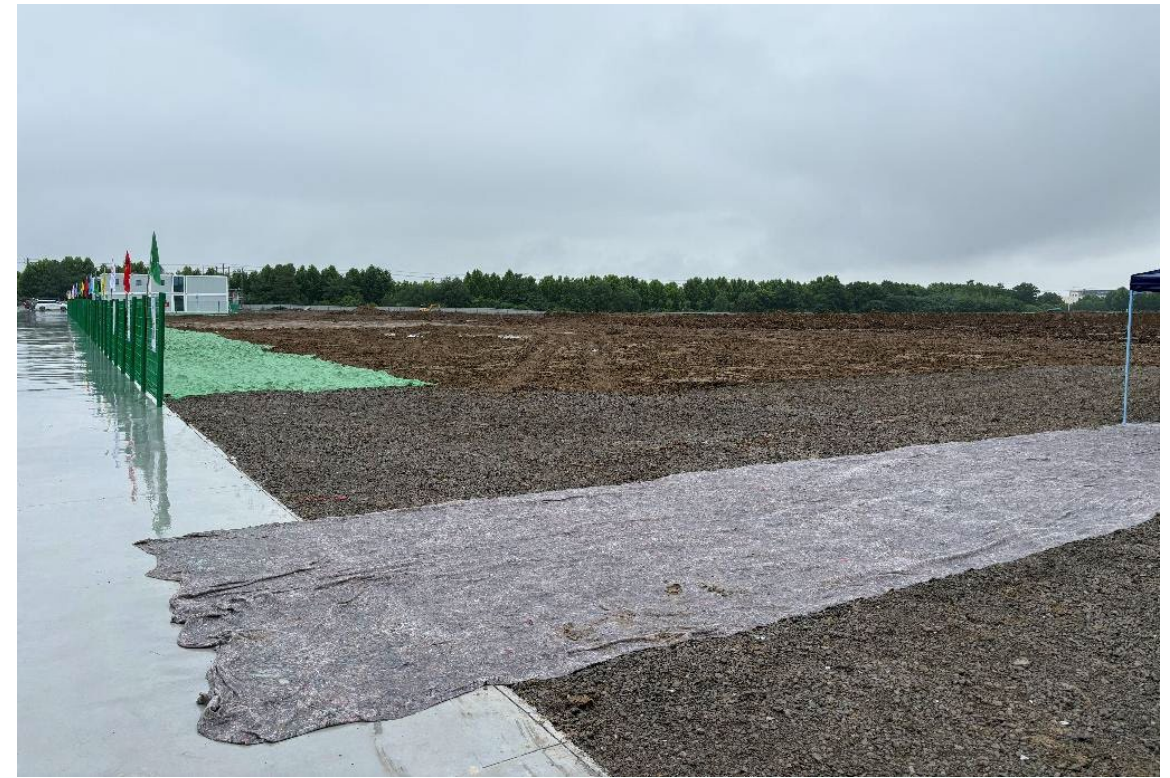
Site planned for factory construction
