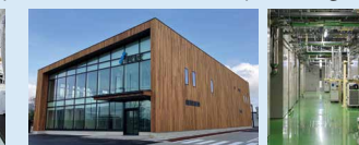
Minami-Alps Plant (Minami-Alps City, Yamanashi) Built in March 2025 Manufacturing base for large-scale production of new etching materials, etc.
